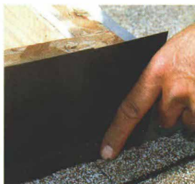
Properly layered flashing and shingles drain the rain. Both the bottom and step flashings are slipped under the shingles. To ease reroofing, flashing is nailed only to the roof deck.
