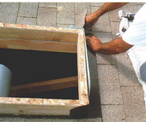
Properly layered flashing and shingles drain the rain. Both the bottom and step flashings are slipped under the shingles. To ease reroofing, flashing is nailed only to the roof deck.
