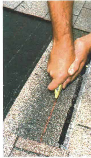
Nails from below show where to snap lines (left). A razor knife with hook blade cuts shingles without harming tar paper (center).
